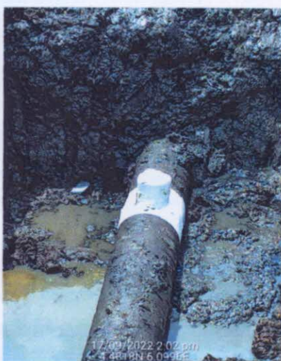
FIG 2-3: Incident Facility repaired and Aqua wrapped
