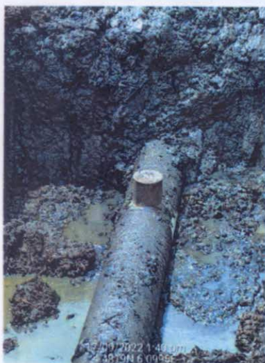
FIG 2-3: Incident Facility repaired and Aqua wrapped
